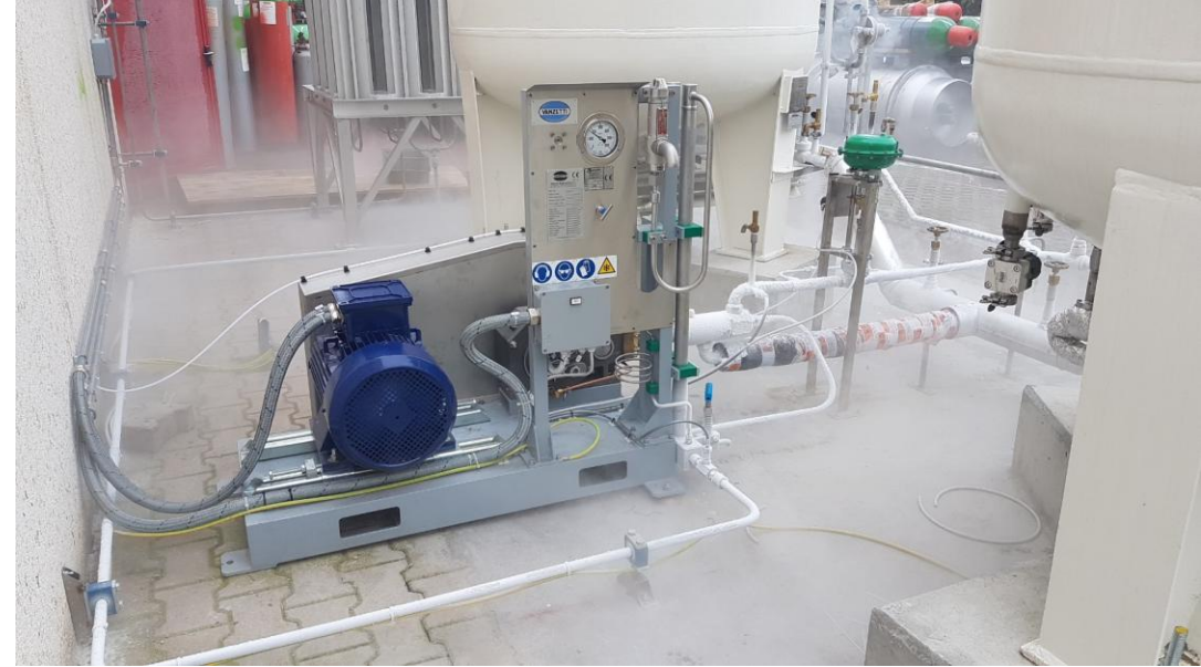
Cryogenic pump Max working pressure: 380bar
